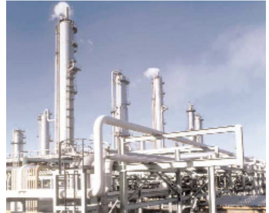
Figure 1: Catalytic reformer in a refinery
